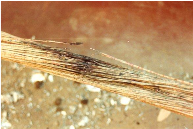
Photo 2: Damaged Telecom Cable
