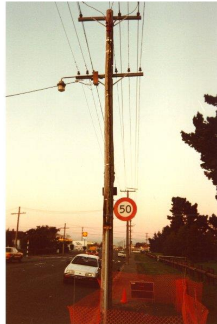
Photo 3: 11 kV Cable on Pole
